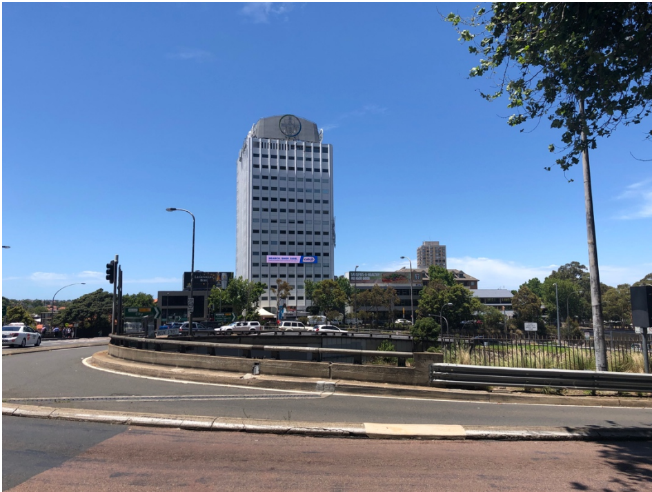
Figure 4 – View of precinct from the west Source: Grimshaw
